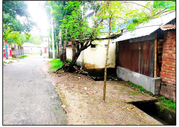
Drain- 01, Kumarkhali Pourashava
