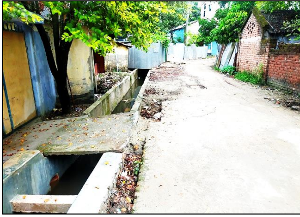
Drain -01, Kumarkhali Pourashava
